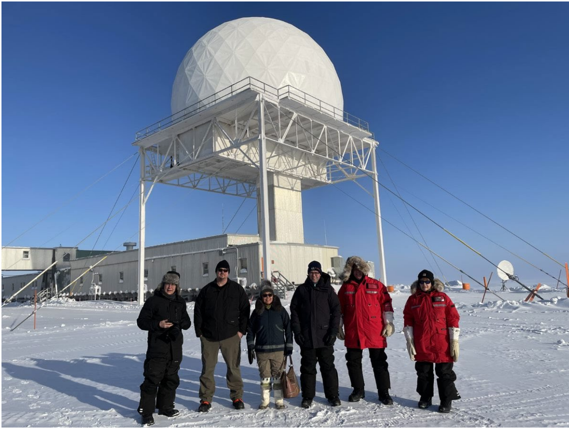
Figure 2—Members of the committee visit the North Warning System in Cambridge Bay, Nunavut
